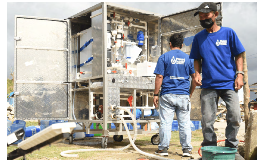
Planet Water Foundation Employees installing AquaBlock water system
