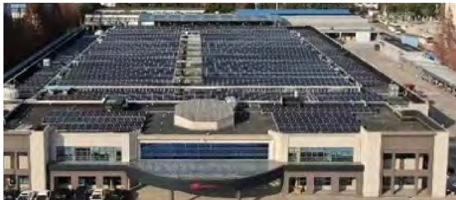
Changzhou, China site, after solar panel installation
