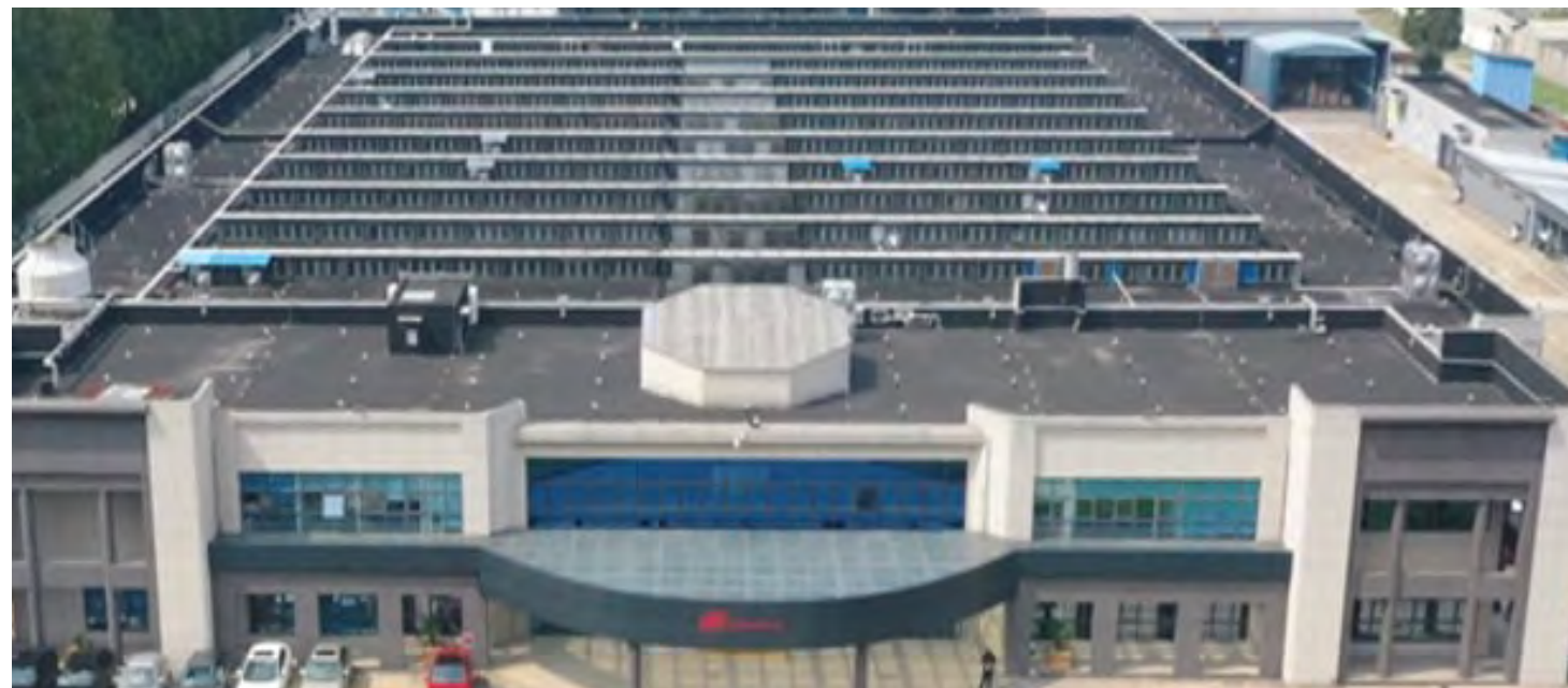
Changzhou, China site, before solar panel installation
